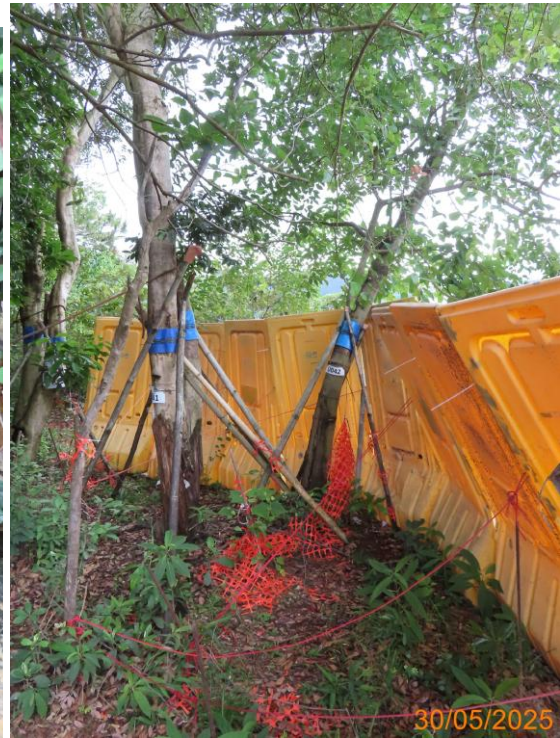
6: Temporary protective fencing for U041, U042 and U043
